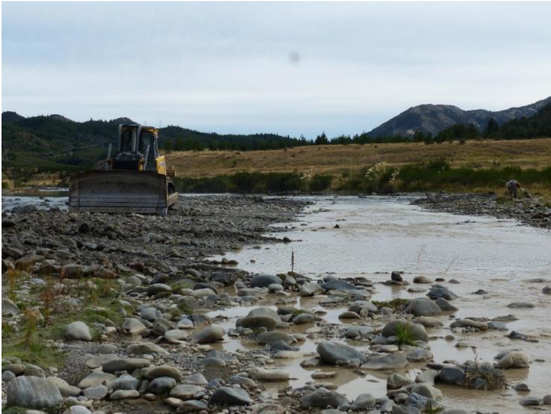
Figure 2.1: An example of island engineering works carried out to improve nesting habitat quality for black-fronted terns on the upper Clarence River. The channel to the right of the bulldozer has been deepened, and the excavated material spread across the top of the island on the left-hand side of the photo, both to raise the height of the island and to bury the woody vegetation growing on its surface. Source: Bell & McArthur, 2016).
