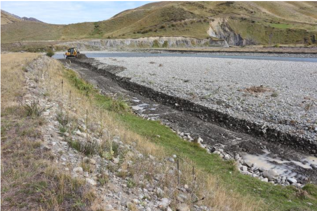
Figure 10. Bulldozer working to open up the newly cleared and deepened channel at upper Bush Gully.
