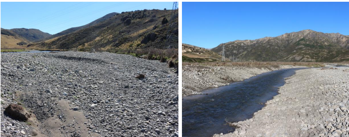
Figure 3. Before (left) and after (right) shots of river gravels blocking channel (left) and channel after being cleared by bulldozer (right).
