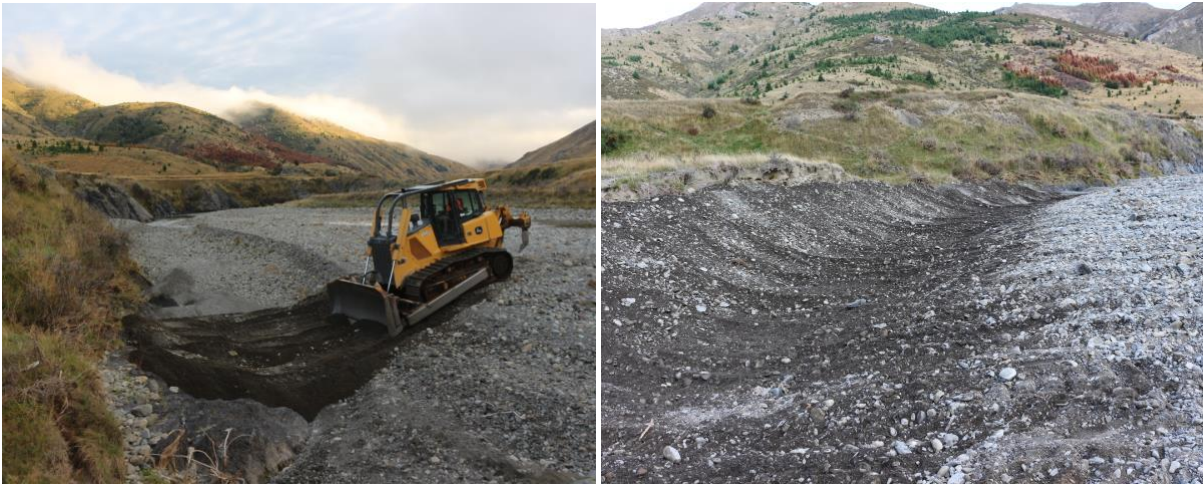
Figure 7. Before (left) and after (right) images of the bulldozer works to deepen and clear channel around the true left side of Eddy's Inlet.
