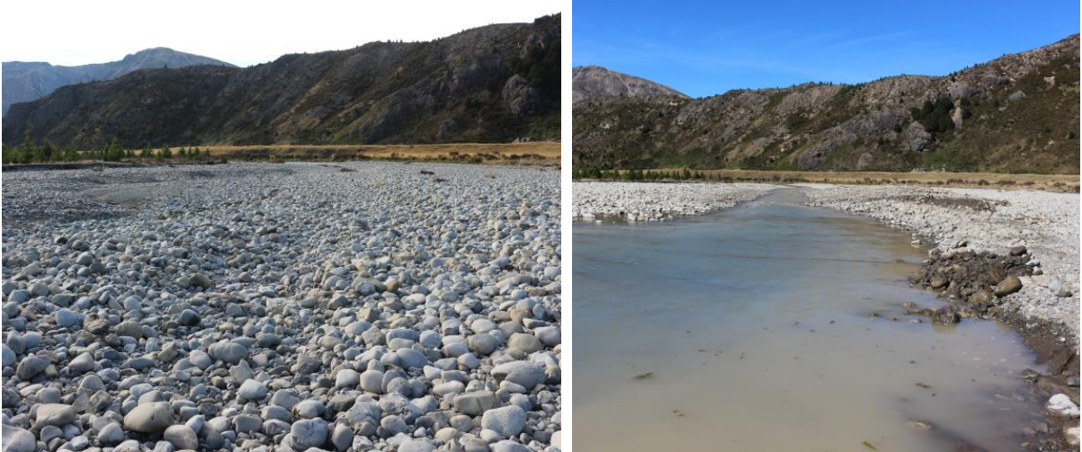
Figure 5. Before (left) and after (right) images of dried up channel along the true left side of Cow Island (left) and bulldozer enhancement works to reopen and clear channel (right).
