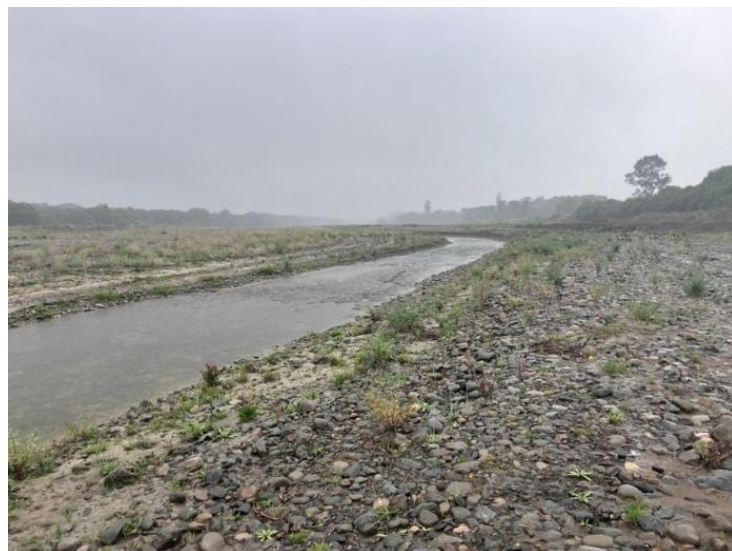
Figure 6: After diversion works on the 16th of January 2026.
