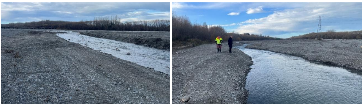
Figure 3: After diversion works are completed, taken 29th of August.
